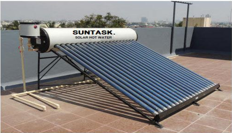
Figure 7: Installed SWH system on rooftop of a house in Hayatabad, Peshawar.
