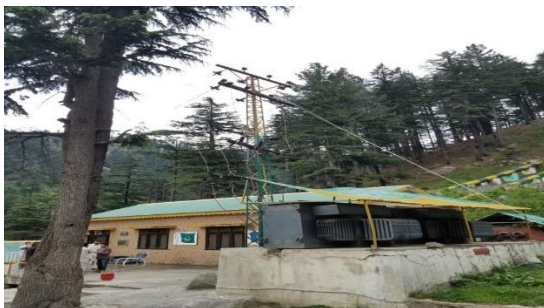
Figure 5. Jungle Inn MHP Project Site view
