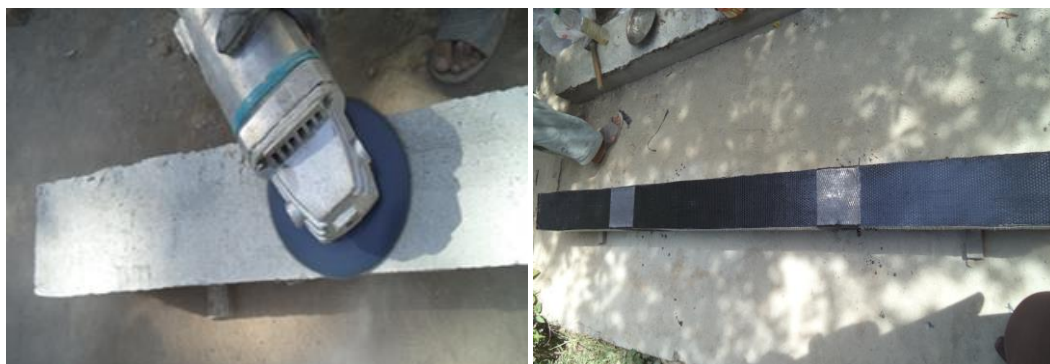
Figure 3. The surface of the beam roughened afore put on CFRP and applied CRFP Sheet on beam
